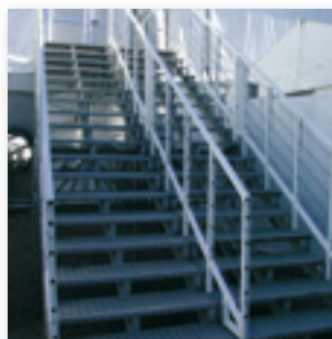
B. STAIRCASE OUTSIDE DOUBLE/TRIPLE DECK STRUCTURE
