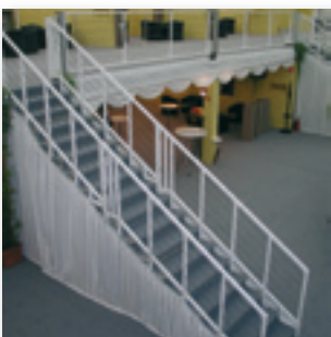
A. STAIRCASE INSIDE DOUBLE/TRIPLE DECK STRUCTURE
